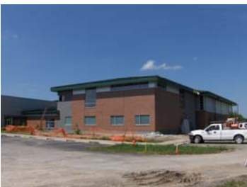
New addition to the Maryville Community Center.
