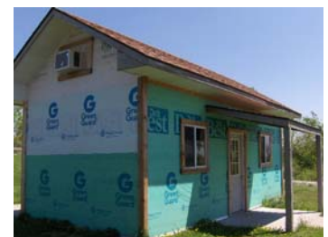
Re-siding a youth cabin
