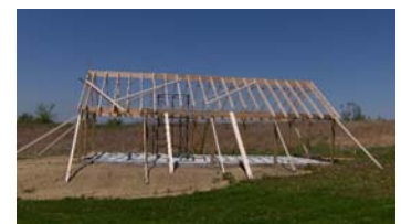
Framing a new youth cabin
