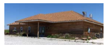
The Multi-purpose building at the Youth Camp
