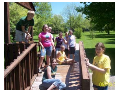
Maryville Middle School volunteers stain the bridge at Judah Park
