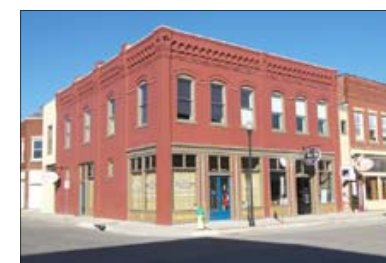
Façade Rehabilitation in Excelsior Springs
